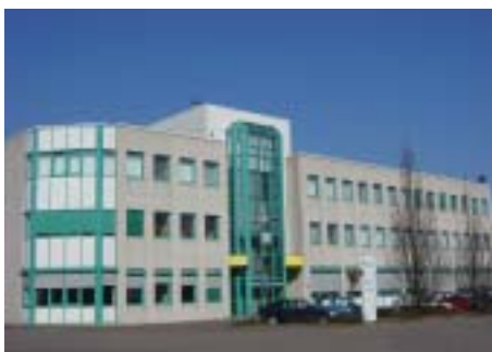
The Dutch company's - Coolmark - head office, which also accommodates a warehouse, is located in Barendrecht, near Rotterdam
