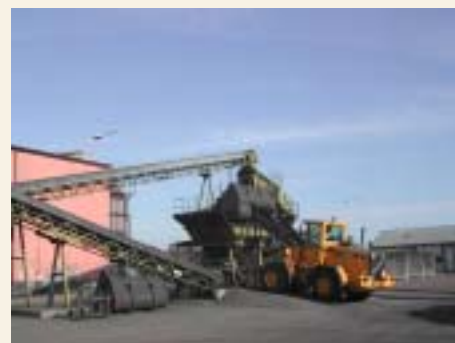
Beijer's coke terminal in Lidköping
