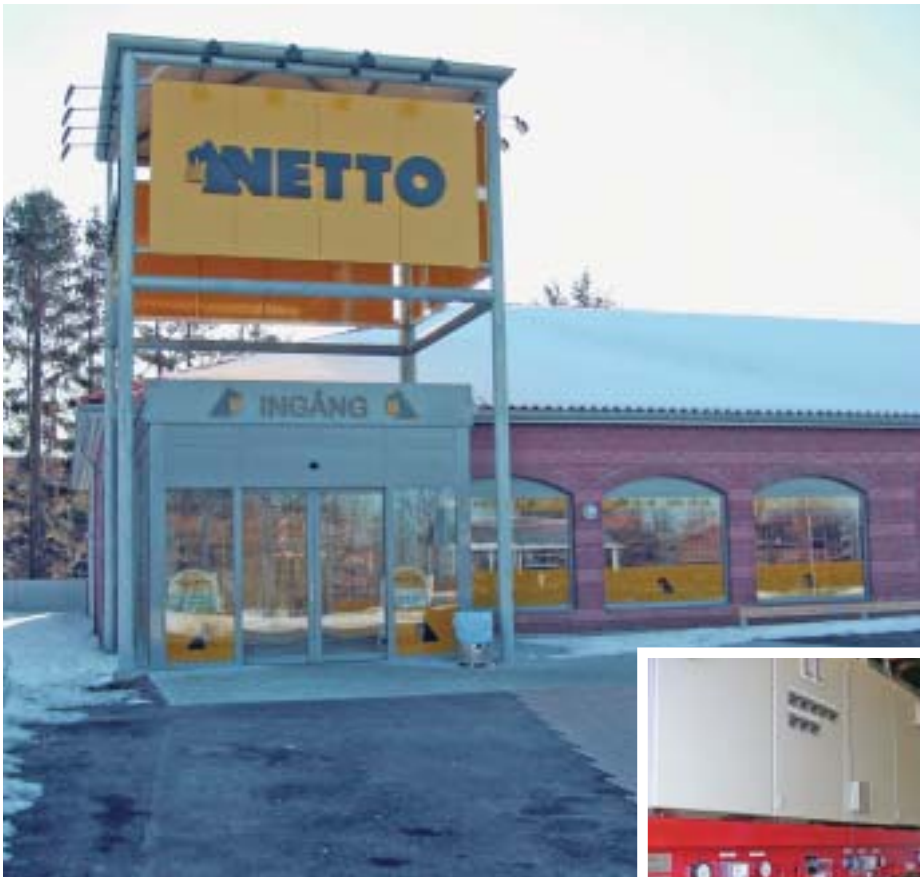
In collaboration with the refrigeration installation company, Hallesåkers Butikstjänst AB, Kylma AB manufactures compressor units which provide cooling for the refrigeration and freezer counters in the Netto food chain. The units are installed in more than 30 stores and an additional 25 Netto stores are planned in Sweden during 2005.
